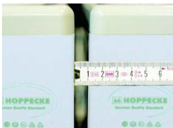
Fig. 5-14: 10 mm clearance between the batteries
