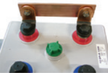
Fig. 5-18: Installing the end terminals (connection plates)
